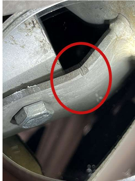
Figure C4 – visible crack on bracket. (Mirror view)
